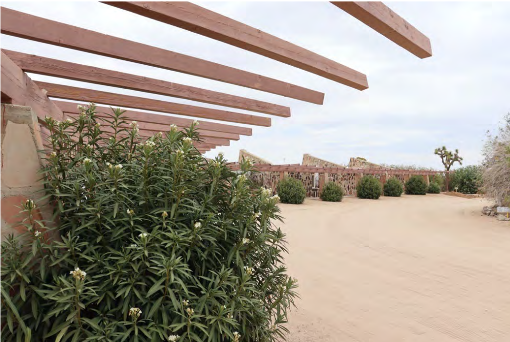
Caravansary of Joy exterior detail. View: N, NE. (CA_San Bernardino County_ New City of Mentalphysics Historic District_0003)
