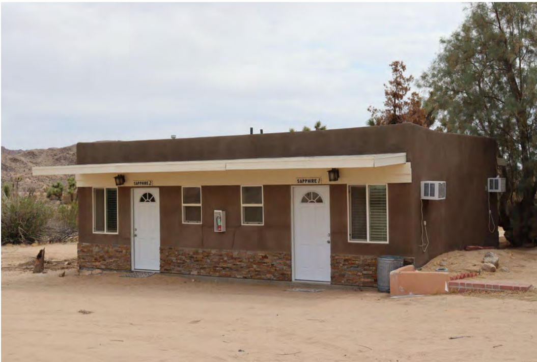
Sapphire Cottage. View: NE. (CA_San Bernardino County_ New City of Mentalphysics Historic District_0042)
