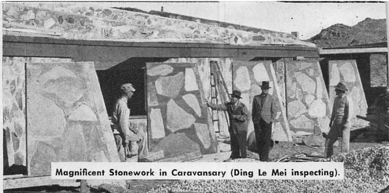
Figure 25. The Caravansary of Joy under construction, 1947. Mansion Builder , Vol. 1, No. 3 (April, 1947), 12.
